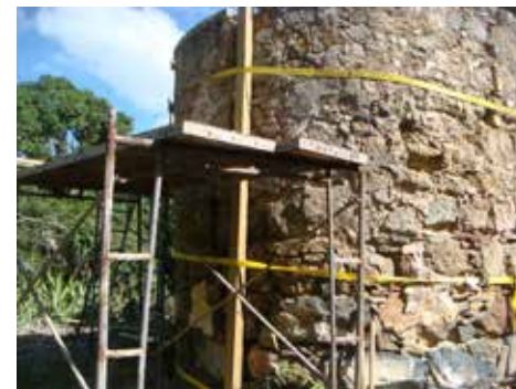
Figure 1 Stabilization of structure
