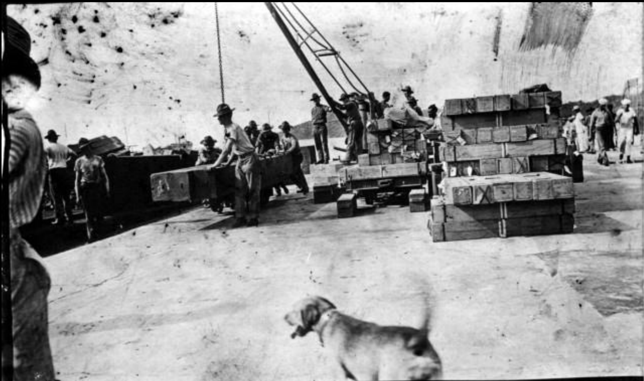
Unloading ammunition and gun mount at King's Wharf.
