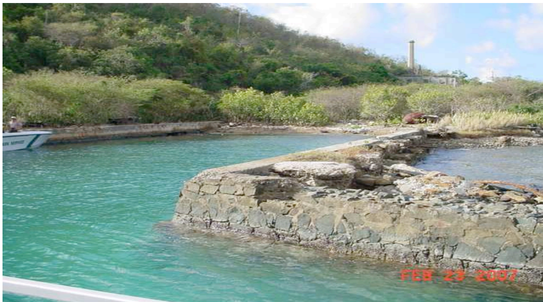
Creque Marine Railway and Head House before
