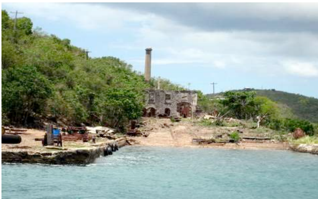
Creque Marine Railway and Head House after clearing
